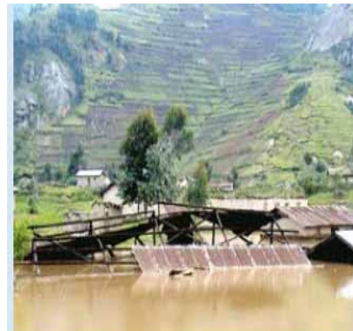
A farm and a house near Gishwati forest damaged by floods
